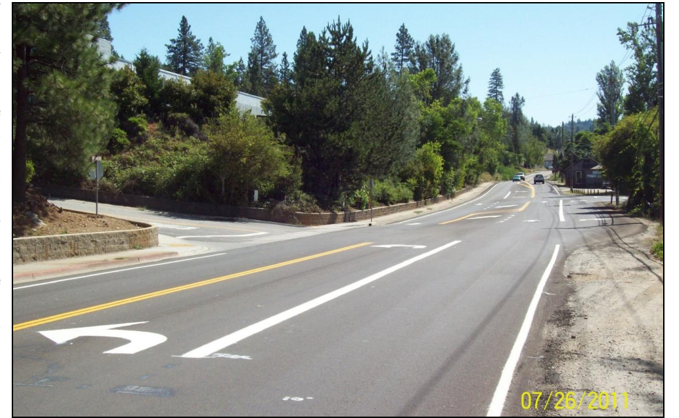
Pavement improvements completed on Idaho-Maryland Road in Grass Valley
