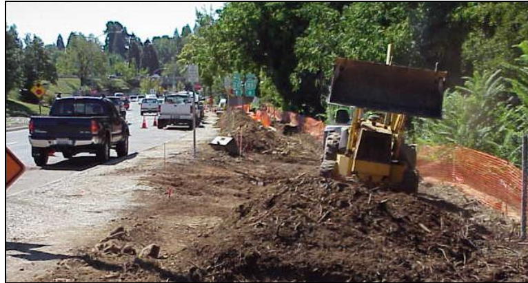
Construction begins on Transit Transfer Center in Grass Valley
